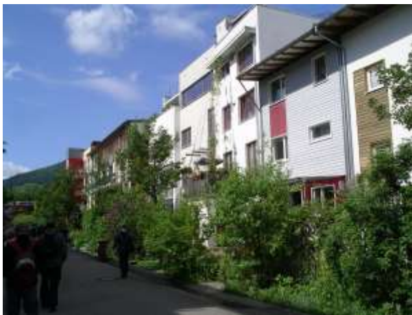
Sustainable family housing, Freiburg
